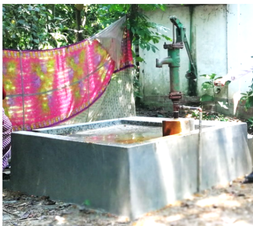
Figure 6-10: Tubewell with elevated platform
