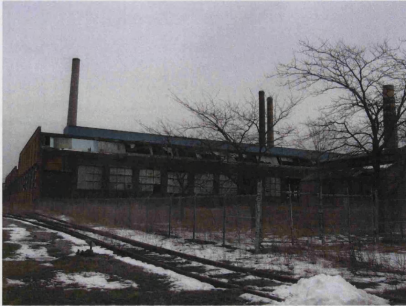
Figure 47 Highland Avenue Brownfield, March 2007.
