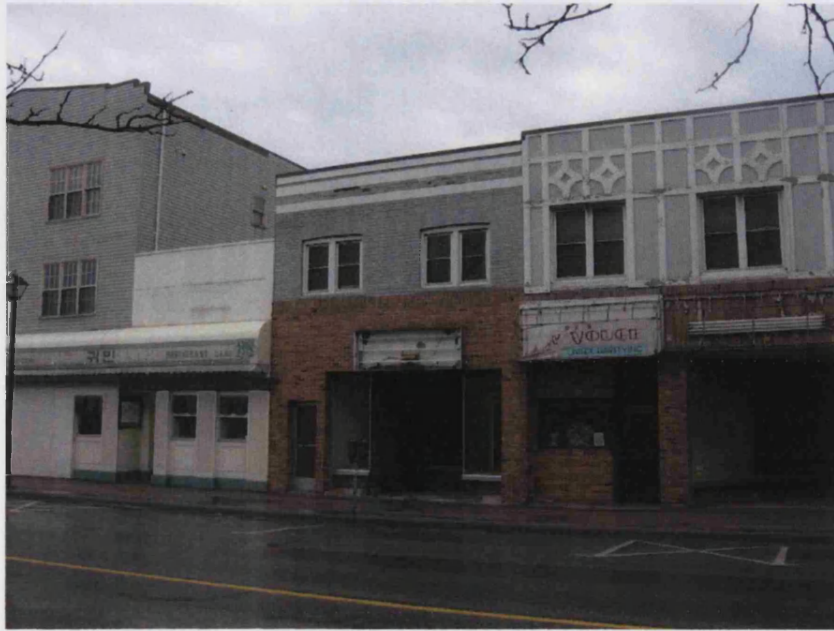
Figure 52 Queen St., Downtown Niagara Falls, Ontario, March 2007.
