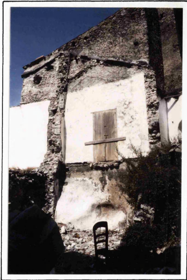
Plate 9.1: Collapsed building in Maratea showing rubble wall construction.
