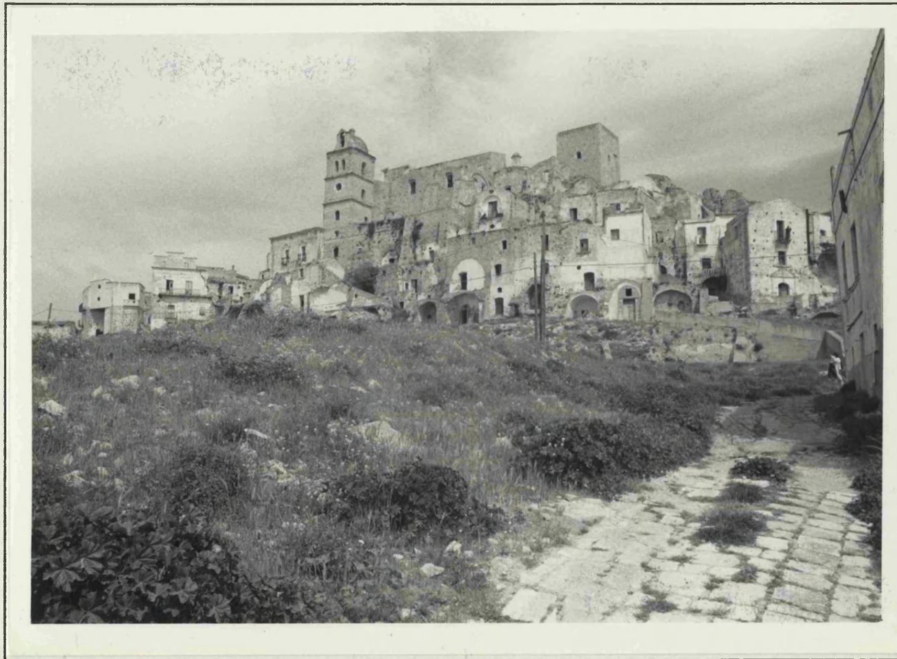
Plate 1.3: The village of Craco in Matera Province, now abandoned because of massive landsliding.
