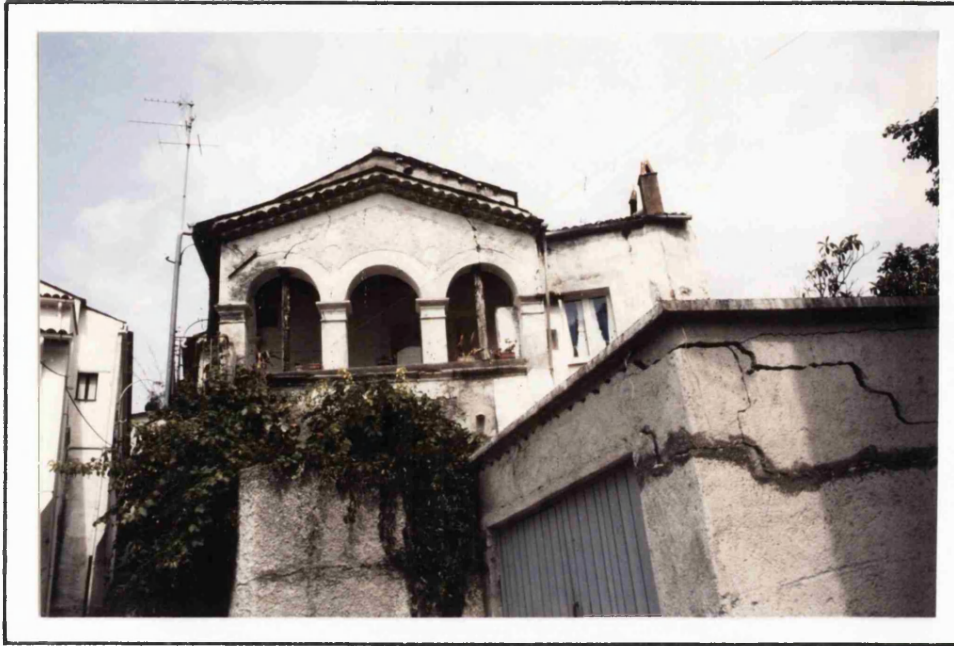
Plate 9.2: Building FG3/163 at the top of the Via Pendinata in the centro storico . The building is seriously damaged (Grade 5), with timber props supporting the balcony arches, yet is still inhabited.
