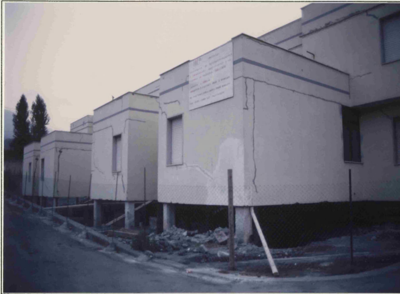
Plate 9.4: Buildings FG4/119 - FG4/121. Constructed in the 1970's, only extensive underpinning has saved these buildings from demolition.
