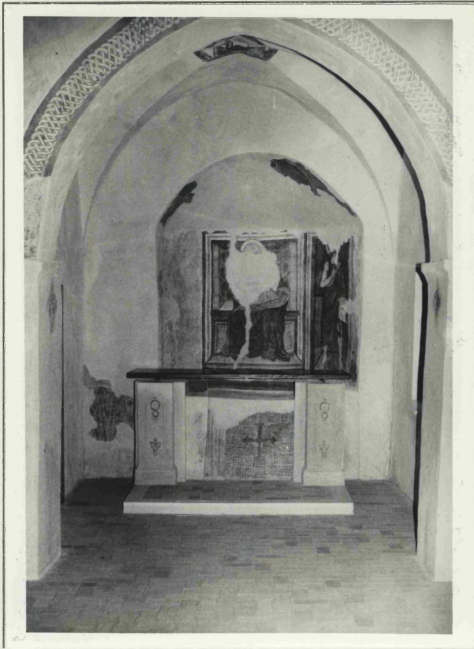
Plate 3.4: Interior of the Chiesa di San Vito - the altar has rotated relative to the main structure. Photograph courtesy of Prof. V. Rizzo, CNR, Cosenza.
