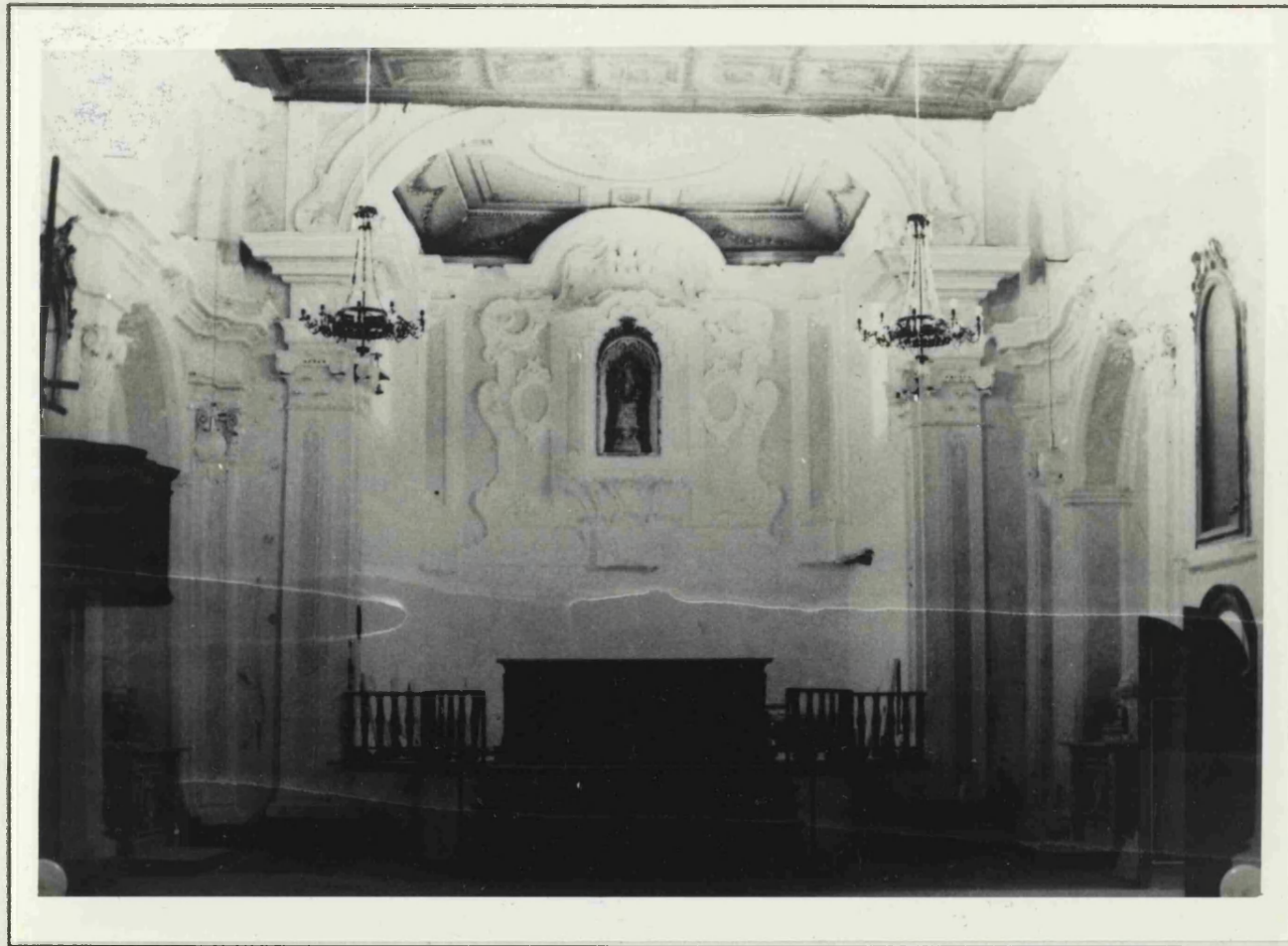
Plate 3.5: Interior of the Chiesa Santa Maria Maggiore - the altar is also thought to have rotated relative to the main structure. The church suffered severe damage during the 1982 earthquake. Photograph courtesy of Prof. V. Rizzo, CNR, Cosenza.
