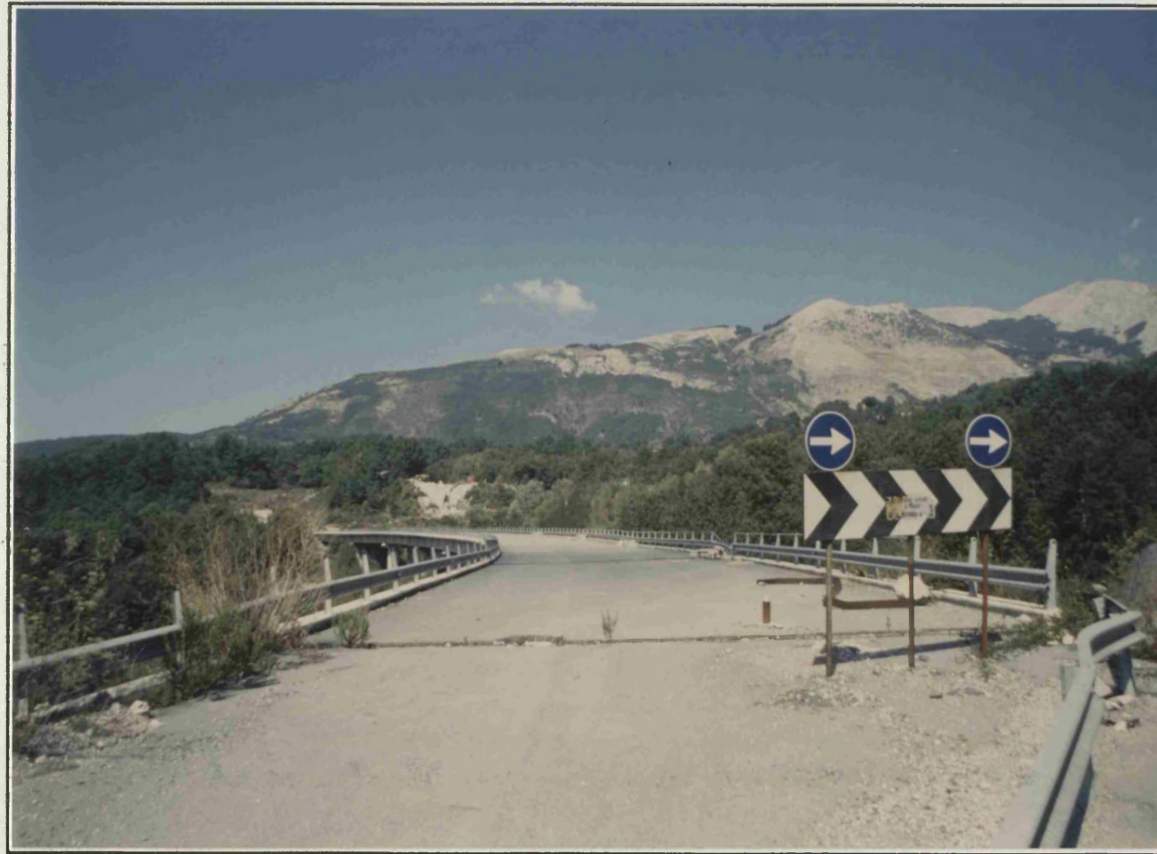
Plate 1.6: Viaduct on the S.S. 92 abandoned due to a rotational landslide. The road was funded by the Cassa per il Mezzogiorno
