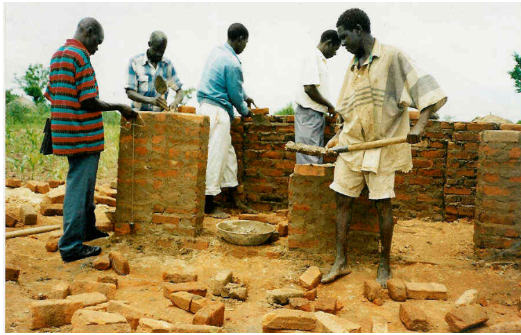
Illustration 5.3 Parents building pit latrines at Cwero (amalgamated) P7 School, 13 April 1999. The bricks were made by parents, the cement bought with parent contributions to the Parent-Teacher-Association (500 Shillings per child).
