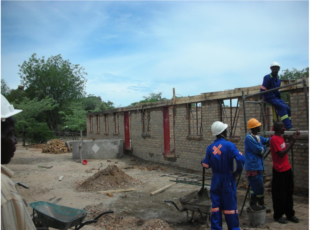
The second of the two planned classroom blocks, under construction.
