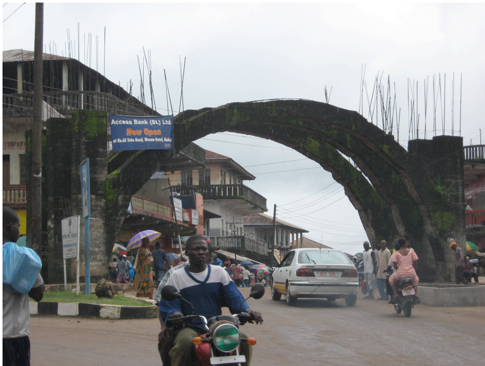
Image 4.1 Makeni's failed clocktower, October 2009 (author's photograph)
